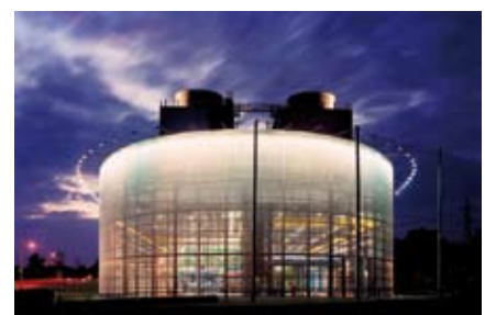
University of Pennsylvania Gateway Complex chilled-water plant, by Leers Weinzapfel Associates Architects, recipient of the 2007 AIA Architecture Firm Award. Photo: Peter Aaron/Esto. Courtesy: Architecture Week
