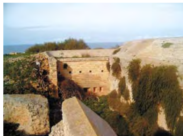
Bomb damage and neglect on outworks of the fort
