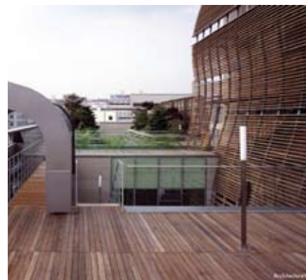
An undulating screen wall composed of steel ribs and wood slats extends through the CHA Women's Hospital. Photo Jong O Kim
