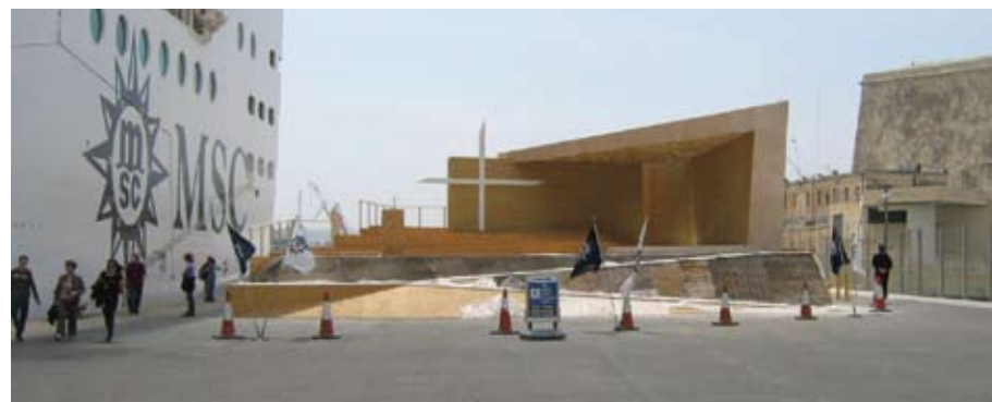
Dwarfed by a cruise liner during construction
