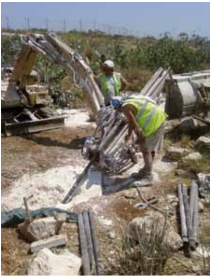
Drilling inclined tension rock anchors
