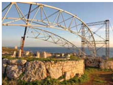
Erection process - note temporary lifting frame
