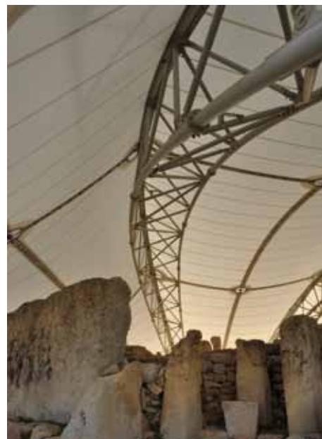
Membrane Roof over Temple ruins
