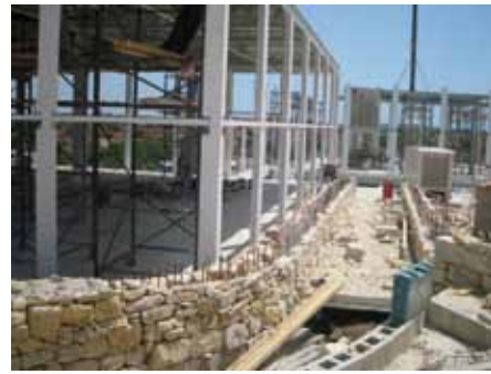
Erection of Visitor Centre
