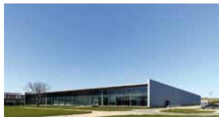
The steel-and-glass Ipekyol Textile Factory in Edirne, Turkey, was designed by Emre Arolat Architects.
