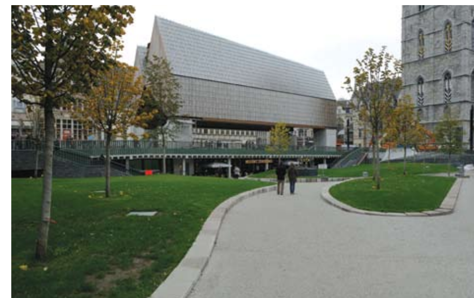
Market Hall, Ghent, Belgium by Robbrecht en Daem architecten; Marie-José Van Hee architecten. Image by Petra Decouttere
