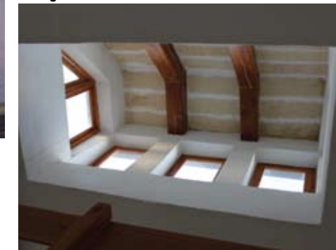
North lights with pivot timber windows at washroom level
