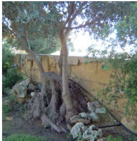
Along part of the Floriana Lines
