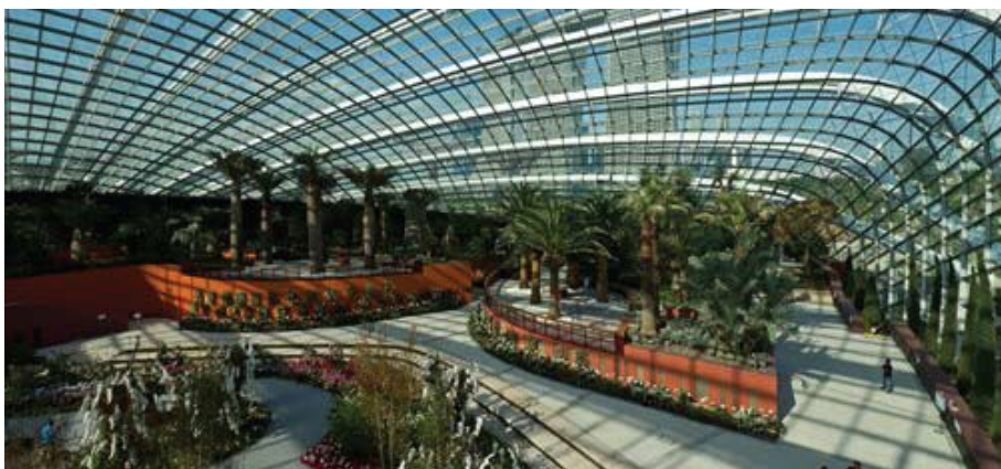
Cooled Conservatories, Gardens by the Bay, Architect: Wilkinson Eyre, Landscape Architects: Grant Associates, Client: National Parks Board
