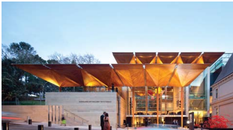
Auckland Art Gallery Toi o Tamaki, designed by Frances-Jones Morehen Thorp & Archimedia.
