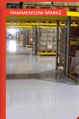
FOODSTUFFS WAREHOUSE MOSTA
