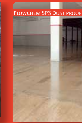
FOODSTUFFS WAREHOUSE LUQA
