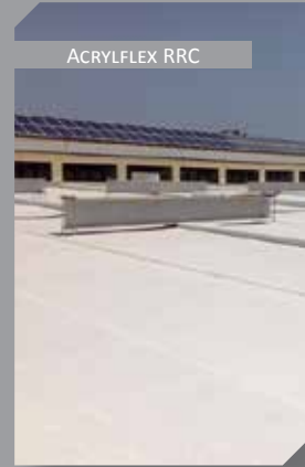
FACTORY ROOF BULEBEL IND ESTATE
