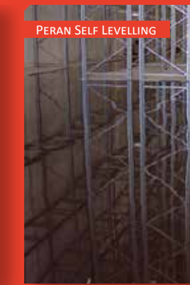
ELECTRONICS FACTORY BUEBEL IND ESTATE
