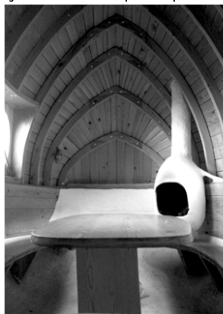
Flying Mud boat tea house - self-built by Professor Fujimori and friends. Built out of timber with cement plaster and copper finish (Japan field trip)
