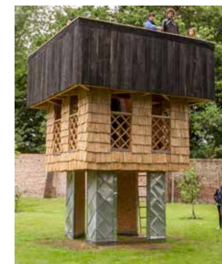
The completed pavilion
