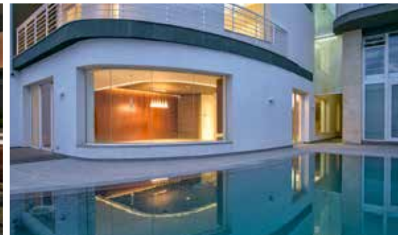
Rapprochement, Zebbug; MJMDA - Matthew James Mercieca Design Architects. Photo by Peter Mercieca
