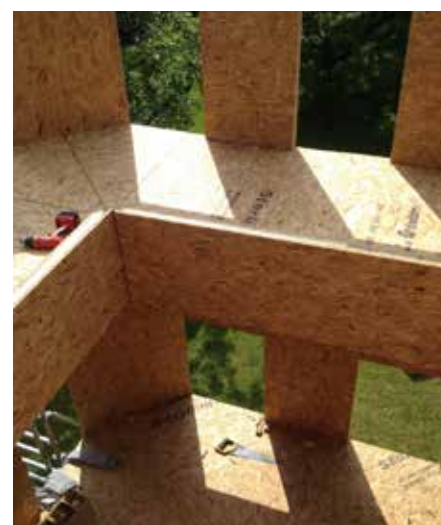
Inner core showing OSB substrate. Table to cover the core allowing users to sit along the edge and dangle their feet (Pavilion construction)
