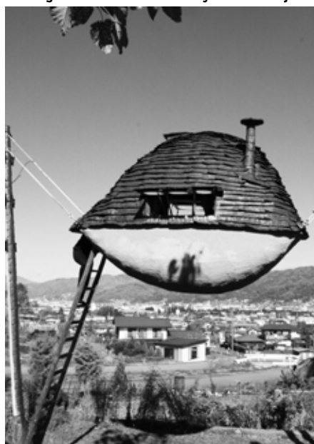
Flying Mud boat tea house - self-built by Professor Fujimori and friends. Built out of timber with cement plaster and copper finish (Japan field trip)
