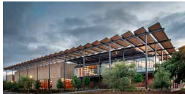
Stanford University Central Energy Facility in Stanford, by ZGF Architects. Photo by Matthew Anderson.
