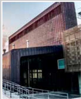
Simonds Farsons Cisk, Copper Cladding
