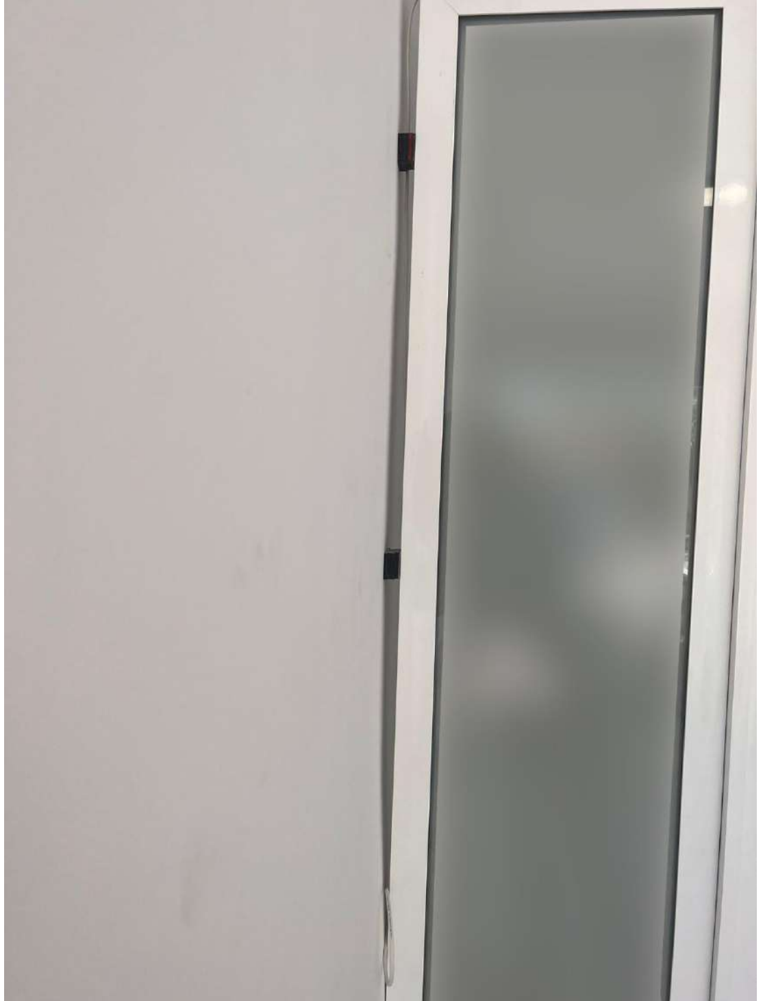
Figure 2 - Door aperture in Qawra. Masonry work and plaster not plumb.
