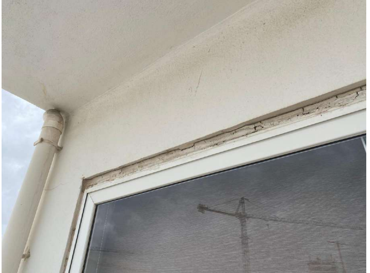
Figure 1 - Door aperture in Gzira. Formwork of concrete beam not laid to falls, resulting in a skewed opening.
