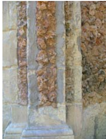
Plastic repair applied to the pilasters
